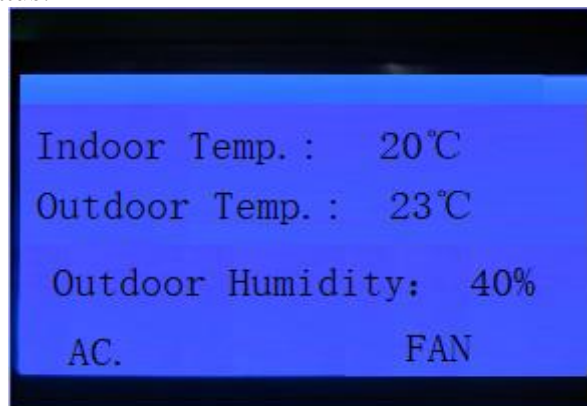
Figure 5. LCD displays the working status of the base station
