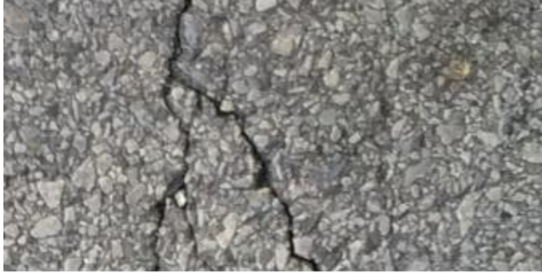
Fig.1 Cracks in pavement
